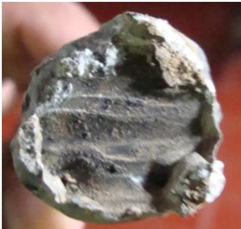
Fig. 4. Visual view of the fracture surface of bolts showing that catastrophic fracture occurred around welded area.
