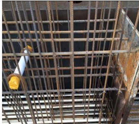
Fig. 6. Embedded parts installation
