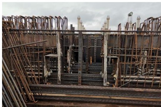
Fig. 7. Steel reinforcement fixing device installation
