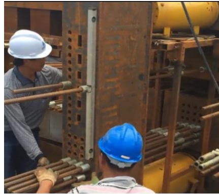
Fig. 9. Overall tensioning of the push jack
