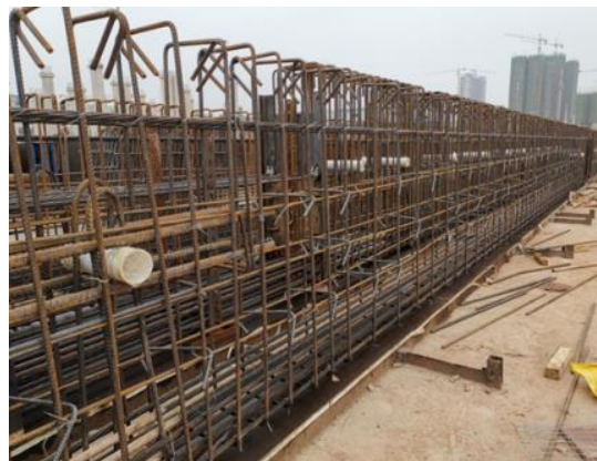
Fig. 5. Steel bars installation
