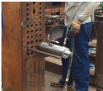
Fig. 8. One-by-one steel strands of the feed-through jack
