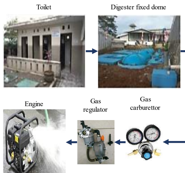
Fig. 2. Biogas system installation
