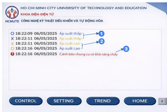
Fig. 10. System Alarm screen (1: Low pressure, 2: High pressure and 3: Warning: Possible fire in the apartment building)
